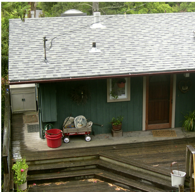
Figure 12. The wide overhang on this home protects the exterior wall from rain. Since many water-related problems in buildings can be traced to leaks at penetrations in the exterior wall (e.g., at windows and doors), limiting exposure would reduce the occurrence of water-related problems. Photo: Stephen L. Quarles.
