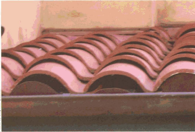
Photo by Stephen Quarles Properly placed bird stops at the end of clay barrel-type roofing can limit the entry of burning embers into the area under the tiles. In this case, dislodged bird stops significantly increases the vulnerability of this roof.
