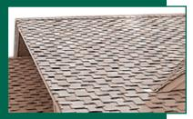
Figure 5-2: Reinforced asphalt shingles
