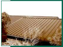
Figure 5-4: Metal roofing
