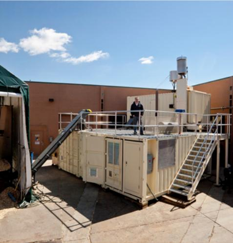
**The modular combined heat and power (CHP) system** on the left will generate 100 kilowatts of electricity and provide 400,000 Btu/hr of heat. The system consumes 2.5 tons of wood chips per day (roughly the equivalent of a rounded pick-up truck load) and provides enough electricity to support a facility such as a school building or recreation center.
