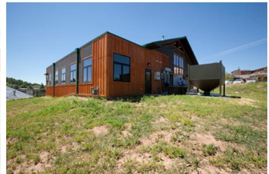
**2010 Colorado State Forest Service Office.** A small 150,000 Btu/hr wood pellet boiler heats this 3,700 ft<sup>2</sup> office building. It is fully automatic – bulk pellets only need to be delivered a few times a year.
