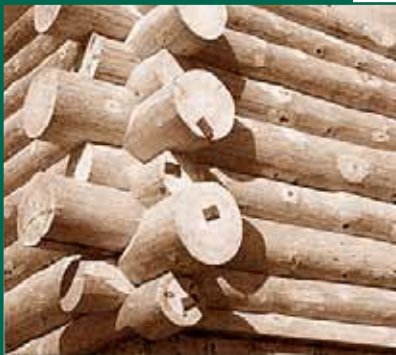
Figure 5-7: Log wall construction
