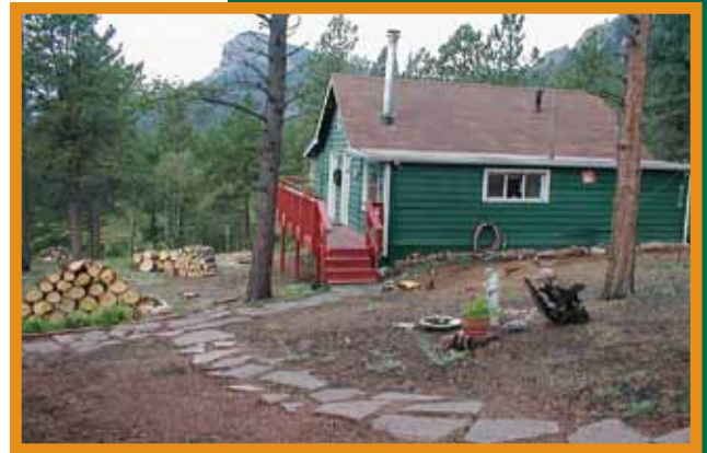
Figure 12: Homesite after creating a defensible space. Photo: CSFS
