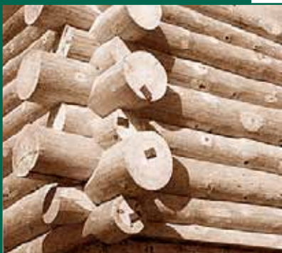
Figure 5-7: Log wall construction
