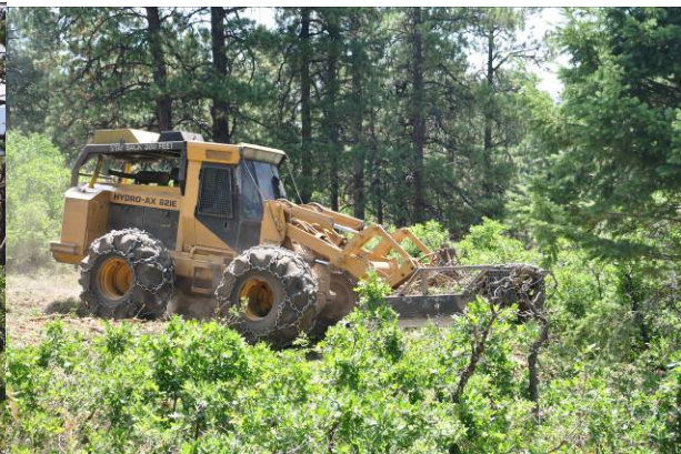
Hydro-axe on the project
