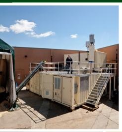
The modular combined heat and power (CHP) system on the left will generate 100 kilowatts of electricity and provide 400,000 Btu/hr of heat. The system consumes 2.5 tons of wood chips per day (roughly the equivalent of a rounded pick-up truck load) and provides enough electricity to support a facility such as a school building or recreation center.
