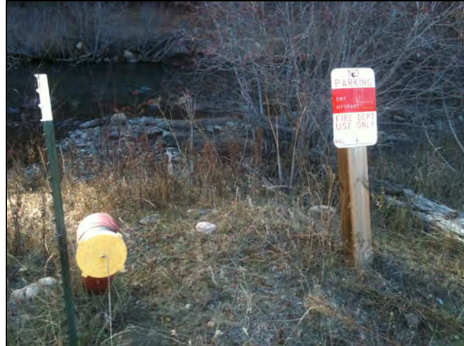
Figure 1. Drafting point (dry hydrant) near Longview
