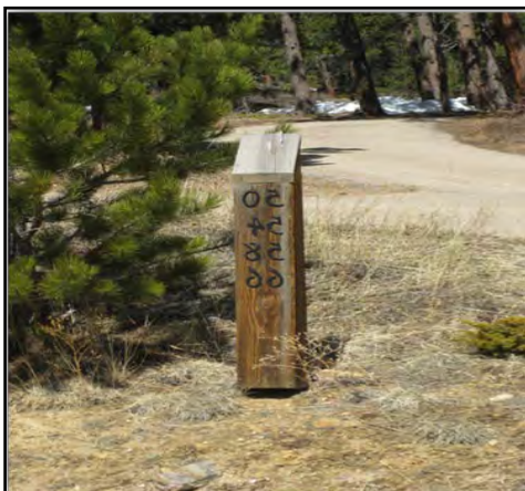
Figure 10. Non-reflective and combustible home address marker with numbers placed backwards.
