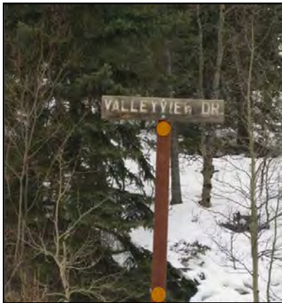
Figure 7. Combustible and difficult to read road sign.
