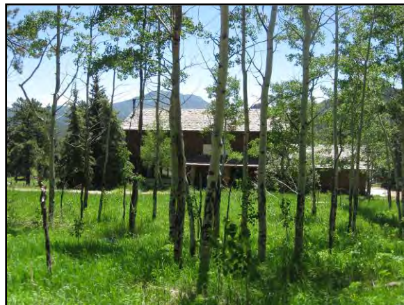
Figure 57. Typical homes in Porter Ranch/Twin Sisters area. Homes are lacking defensible space and many have combustible wood siding.
