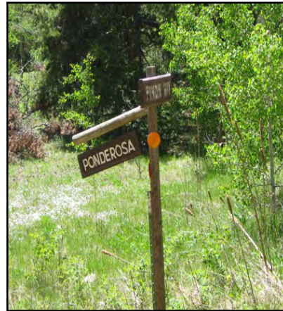
Figure 8. Combustible and non-reflective road signs.
