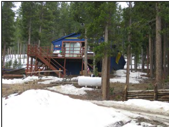
Figure 15. Home with combustible deck and open area under the deck.
