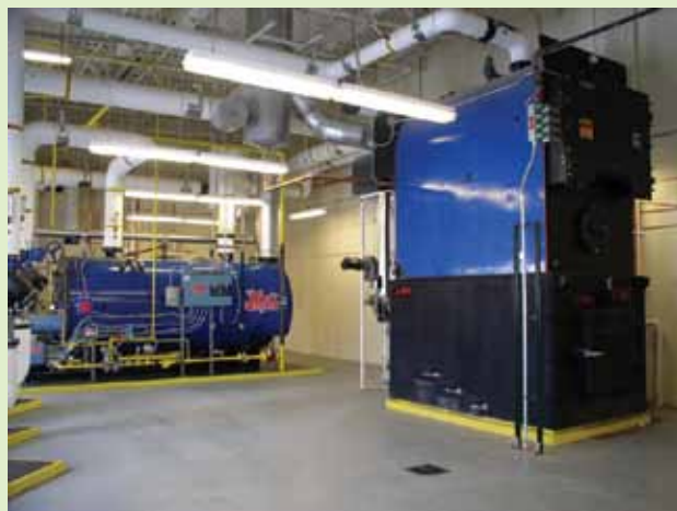
Biomass furnace that burns chips and heats county facility
