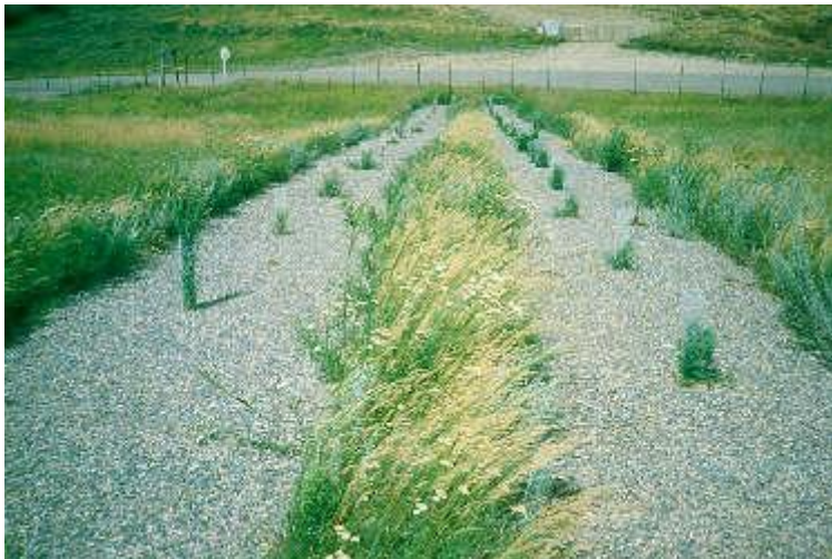
Fabric with gravel on top
