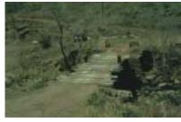
■ Roads, driveways and bridges should be built to carry at least 40,000 lbs., the average weight of a fire engine. (By comparison, the average family station wagon weighs about 4,000 lbs.)
