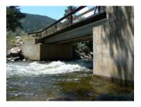
Crown Point Dr & U Bar U lane – To access these roads you need to cross a bridge made with concrete supports and wooden decking. The bridge was is safe to handle all current PCFPD trucks. Recently the bridge has supported a concrete truck carrying about 6 yards and also a well drilling rig.
